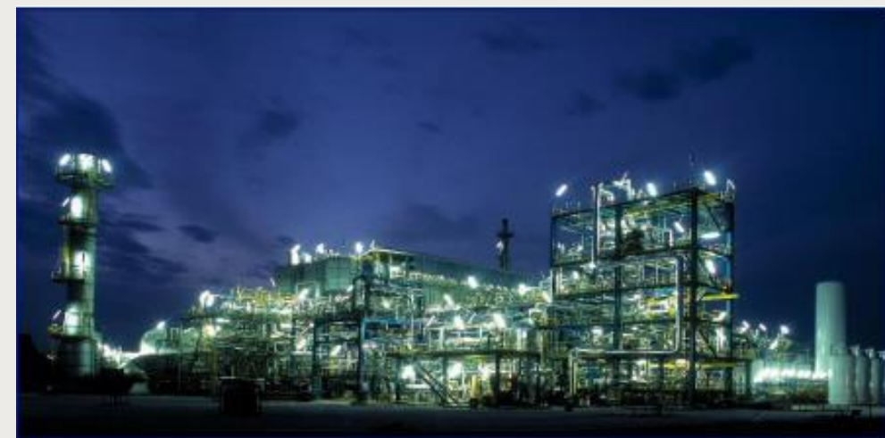
Air Liquide, Port Jerome (SMR +CCS)
