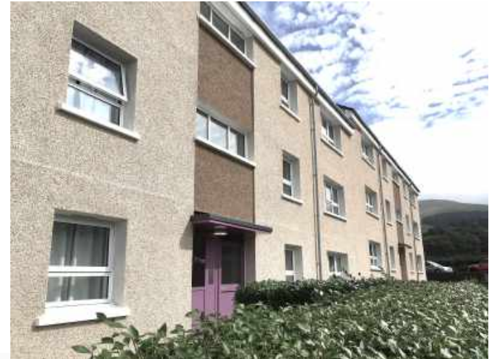
Refurbished block for Ayrshire Housing, Rowan Road, Girvan,
