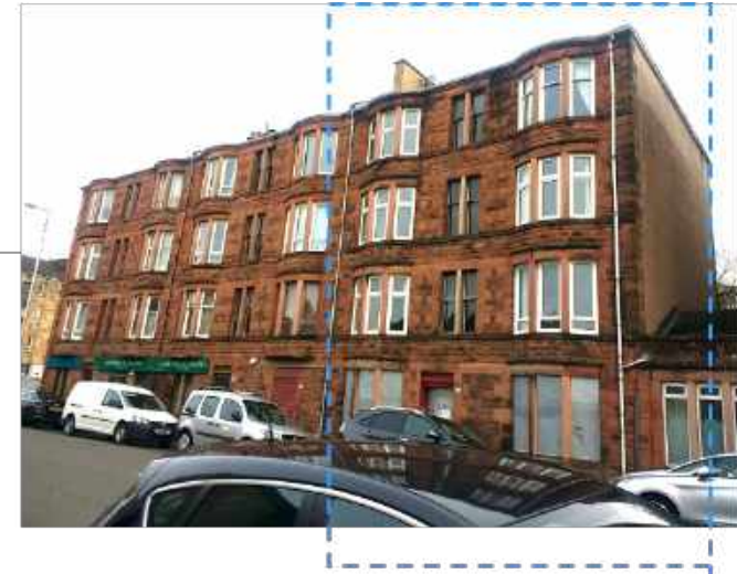
Niddrie Road Enerphit: John Gilbert Architects
