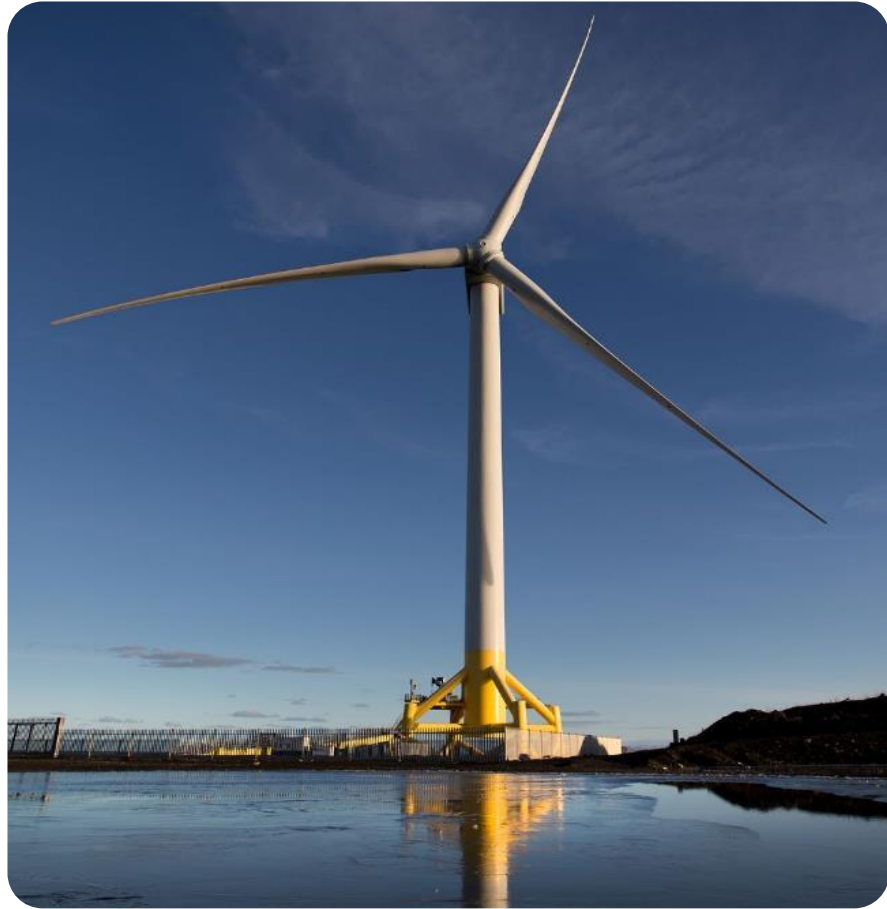
ORE Catapult 7MW Turbine
