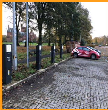
EV Charger installation and maintenance
