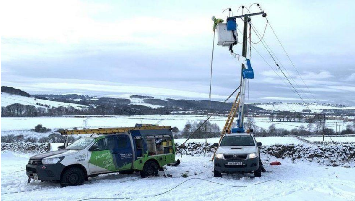
Image: Electricity North West https://www.bbc.co.uk/news/uk-59396135
