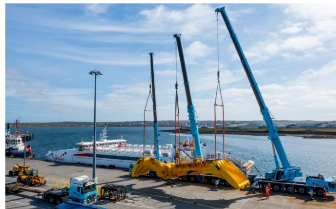
Mocean crane lift on Hatston Pier by Heddle, Orkney. Photo: Colin Keldie
