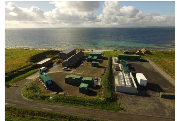
EMEC Caldale substation and hydrogen plant (Credit Orkney Sky Cam, courtesy of EMEC)
